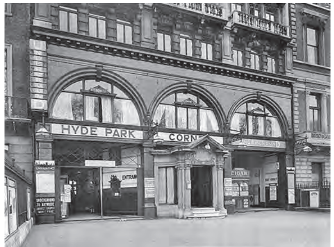
Hyde Park Corner station entrance in 1925
